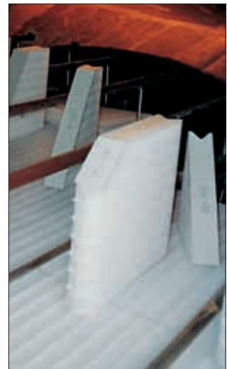
LTV 271 during installation
