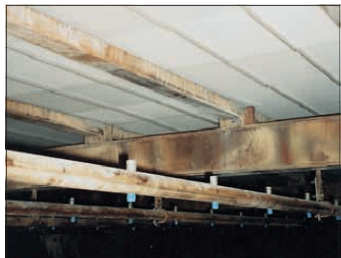
Installed LTV 400 in a flue-gas desulphurization plant
