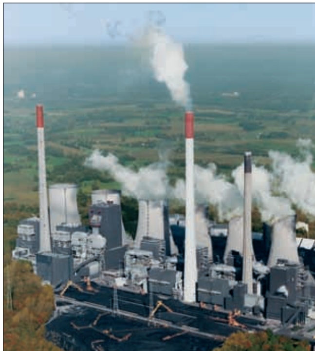
Power plant (EON)
