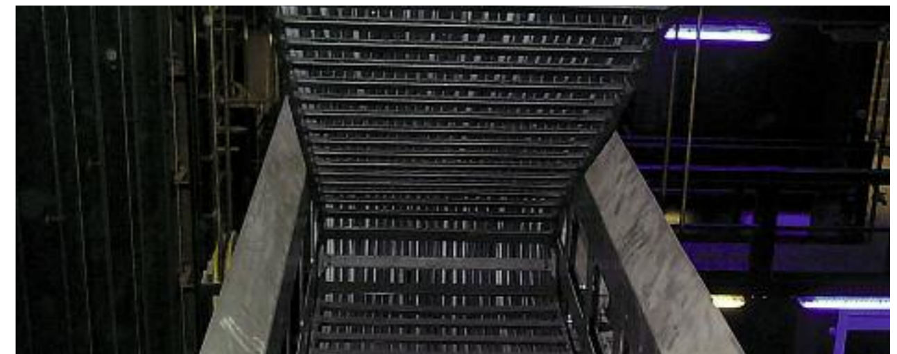
Coax cables and other chainflex® cables in platform technology. e-chain®: System E4/4
